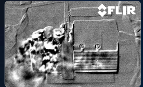
HIGH SENSITIVITY MODE IMAGE OF LEAKING AC UNIT
