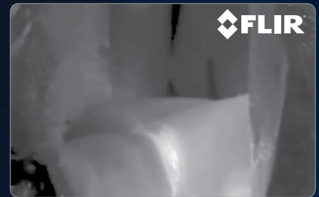
IDENTIFY LEAKS IN VALVES
